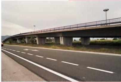
This bridge that crosses the freeway has a length of more than 300 m. It is made with post-stressed concrete provided by PIONEER CONCRETE HISPANIA, which we were its exclusive supplier. In three days it had to give more than 20N/mm<sup>2</sup>. To tighten, a cement of high initial resistance was used.
